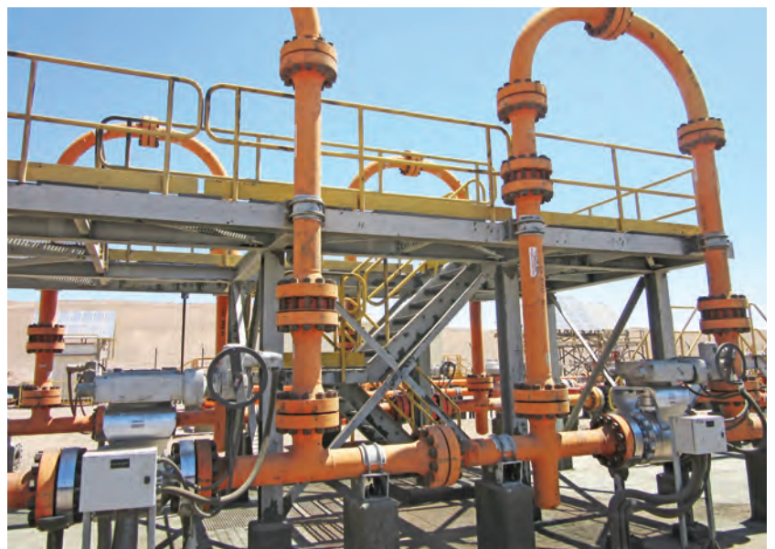
Velan Securaseal C-series valves installed at one of the most severe slurry pipelines in Chile. Velan valves are exceeding the performance requirements in one of the toughest slurry pipelines in the world.
