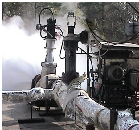
Line break testing (blowdown) (1)
