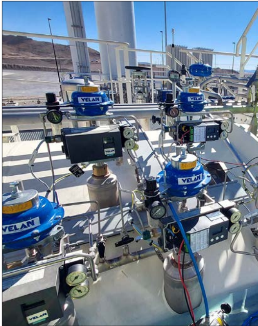
48 Cryogenic angle and straight regulating globe valves installed in a liquid hydrogen production plant located on the west coast of the United States and manufactured by Velan S.A.S., in France.
